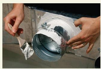
**Tight ducts save money.** Sealing leaky ductwork can be done in several ways, but mastic and fiberglass-mesh tape are among the best options.
