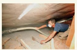
**Pile it on.** If adding rigid foam on top of the roof sheathing isn't an option, a less expensive option is blowing cellulose on an air-sealed attic floor. The more insulation, the better.
