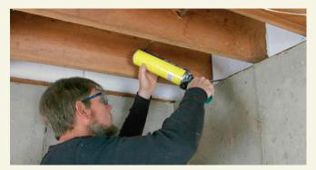
Stop the leaks. If a full basement-insulation job isn't in the budget, attack the rim joist. Spray polyurethane foam works best, but a more affordable option is to seal rigid-foam panels in each joist bay with canned spray foam.
