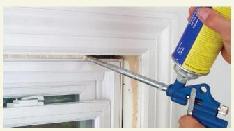
**Air-seal, then insulate.** If you can't afford to add insulation to your walls, address simple air-sealing measures such as filling the gaps around windows, electrical boxes, doors, and recessed lights in the ceilings.
